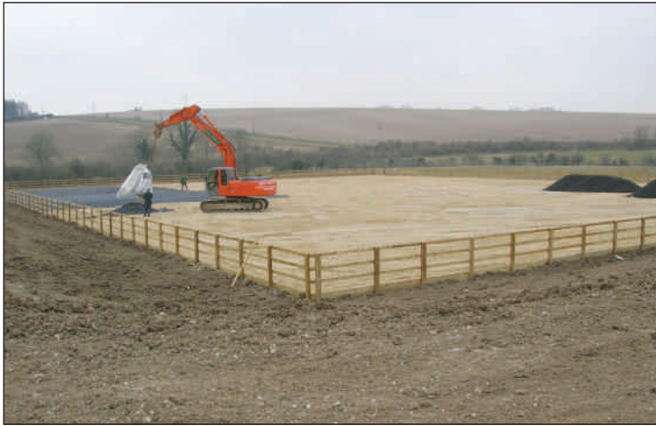
The new 80 x 60 Arena at Escombe under construction
